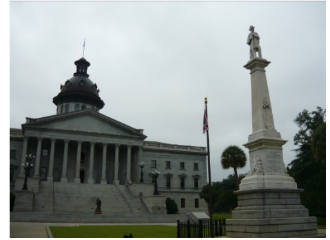
The South Carolina State House and Confederate Monument, 2009: Flagpole and fencing in place.
